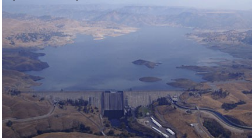
Completed in 1942, the Friant Dam on the San Joaquin River in California is an example of a concrete gravity structure.
