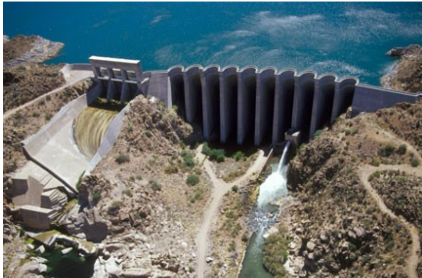
Built in the 1930s, the Bartlett Dam in Arizona is an example of a reinforced concrete, multiple arch and buttress dam; it consists of 10 arches, nine buttresses and two gravity wing dams.
